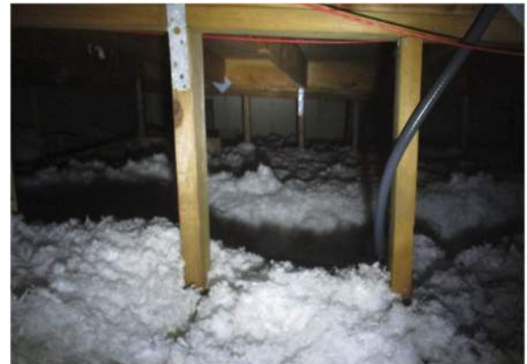
Roof Framing in Attic Space Above Lobby
