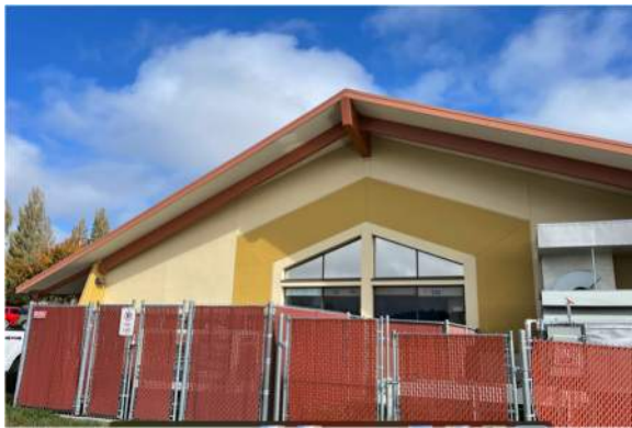
Overall Building View Looking Northeast
