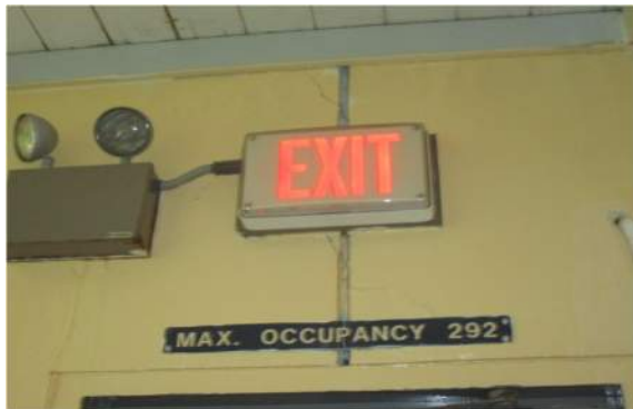
Temperature Cracking over Northeast Exit Door (Interior)
