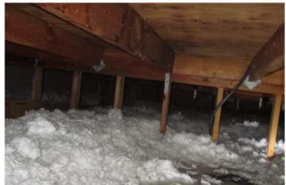
Roof Framing in Attic Space Above Lobby
