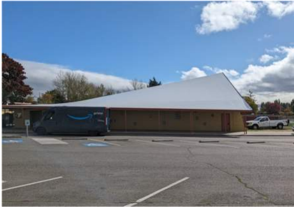
Overall Building View Looking Southeast
