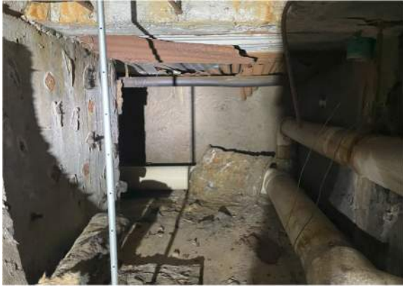
Northwest Ventilation Tunnel Looking Northeast
